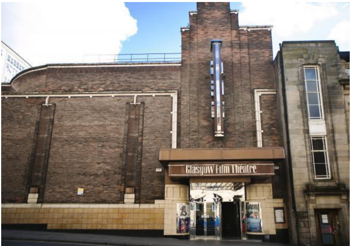
GFT Main Entrance.
